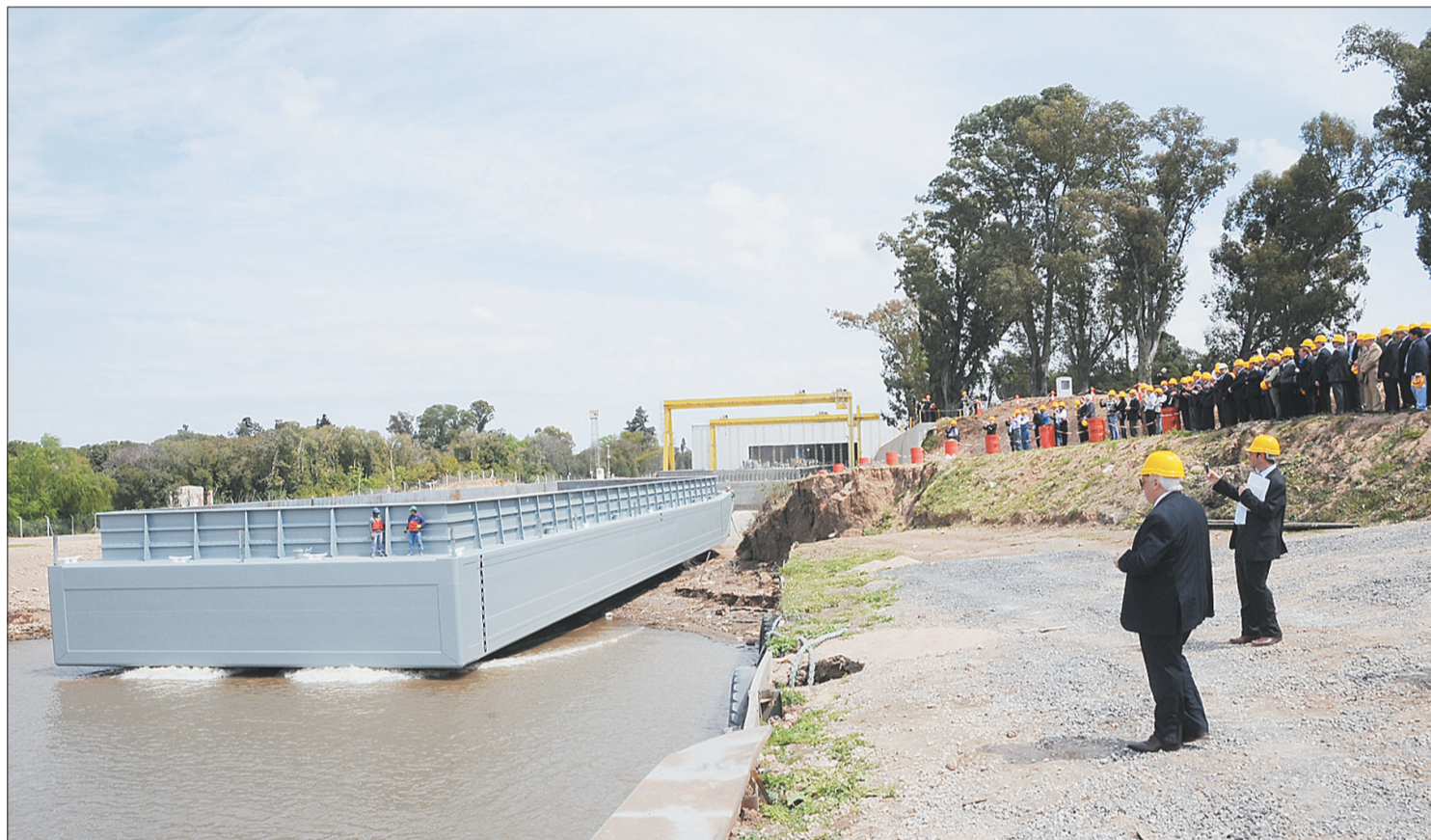
A barge is launched onto the River Paraná by the private Ultrapetrol shipyard on September 27, 2013, in Punta Alvear, Santa Fe Province. (Photo courtesy Willy Donzelli).
